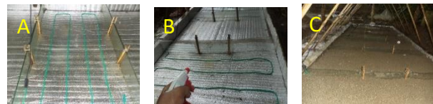
Figure 2. Soil heater installation in the propagation box.
